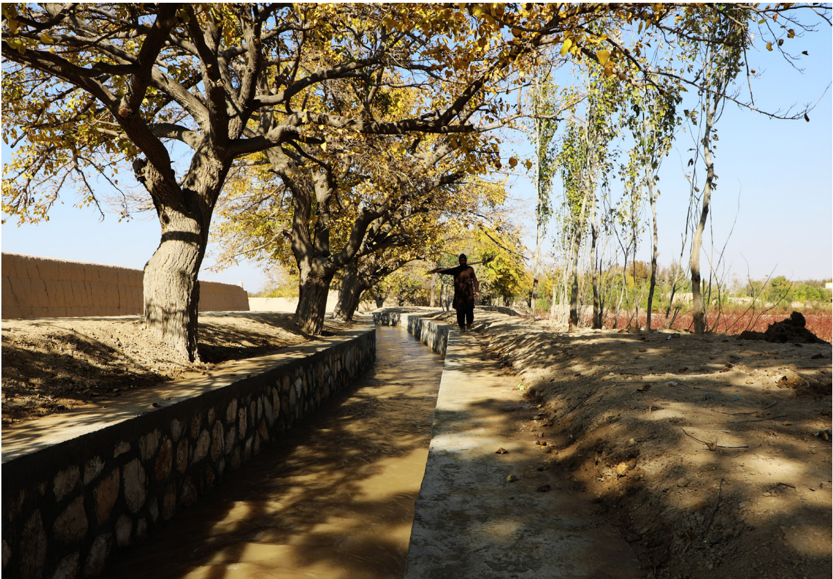
The Langarkhana Canal in Mazar-e-Sharif has become a lifeline for local communities during flash rains. With its strategic location and design, the canal helps divert and manage excess water, preventing flooding and protecting surrounding areas.
