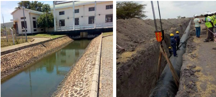
Photo 13: Ongoing Lake Victoria Water Project
