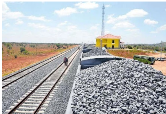
Photo 6: Ongoing construction of a standard gauge railway (SGR)
