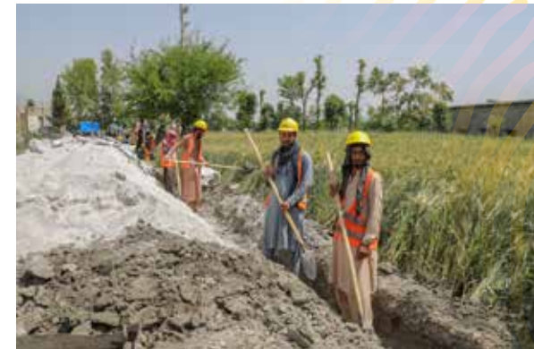
Canal rehabilitation in Nangarhar province, Eastern region
