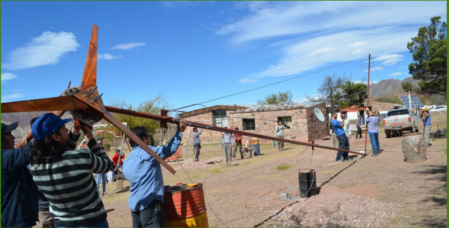
500Rpm, a non-profit organization in Argentina adapts the Piggott wind turbine design to make low-cost renewable energy accessible in rural areas in Latin America. Photo: 500Rpm.
