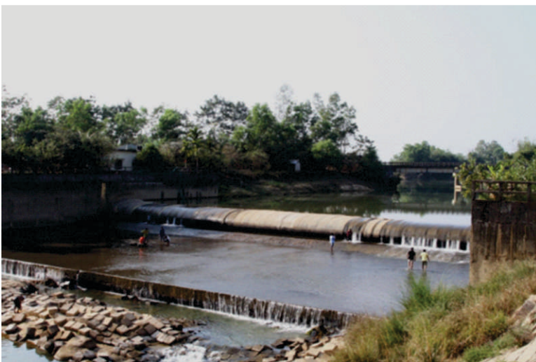
Figure 16: Bhujpur rubber dam in the upstream of Halda River drastically reduces the water supply in the downstream during the dry season
