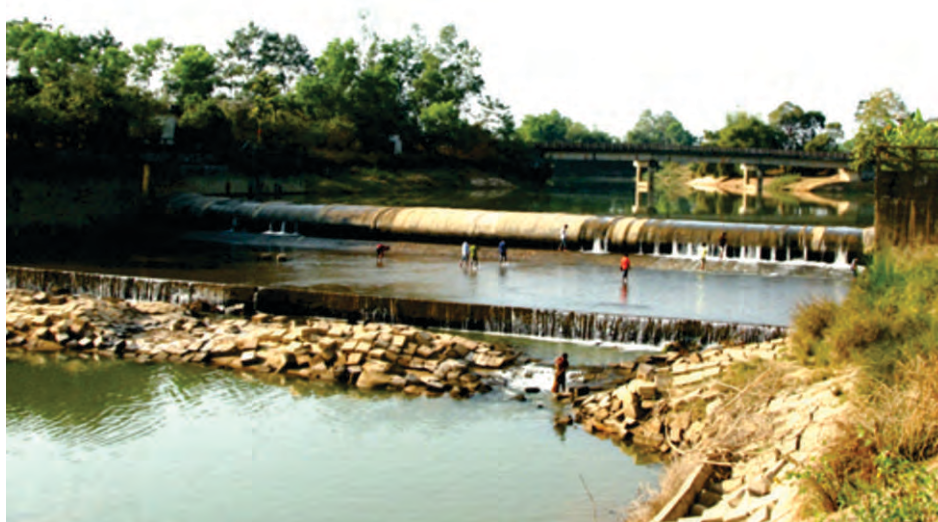
Rubber Dam at Bhuzpur on the upstream of the Halda River (6 th February 2019)
