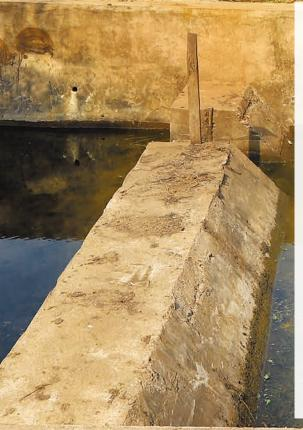
The check dam was approved and constructed under Mahatma Gandhi NREGA. It allows the cultivation of an additional crop (rabi) on one side of the stream, whilst the other side of the stream has been converted to cultivable land from a wasteland. The dam also collects water that enhances the irrigation potential in the region.
