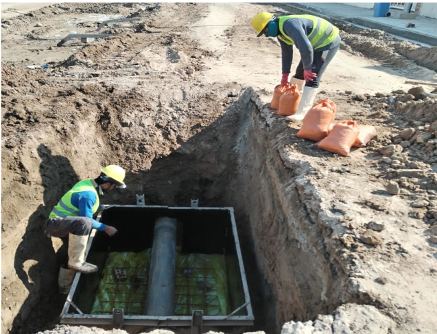
Casting the foundation of the manhole
