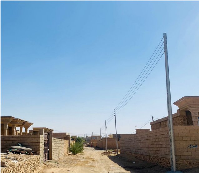
Rehabilitation of Electrical Networks in AlSenia, Baiji
