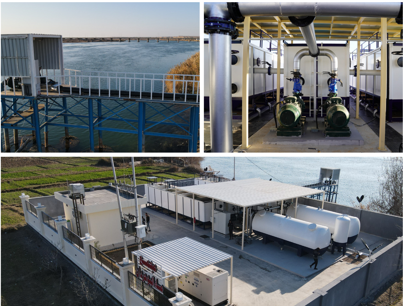
Rehabilitation of Albo-Hardan Water Complex, Al-Rummana, Anbar governorate
