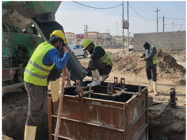
Casting the Walls of the manhole
