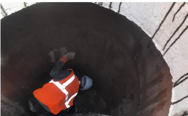
Cleaning the manhole before epoxy painting
