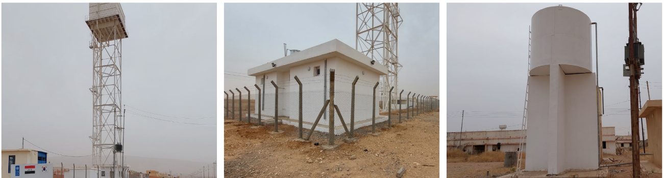
Refurbishment of Water and Sewerage System in Domez Complex, Sinjar, Ninewa
