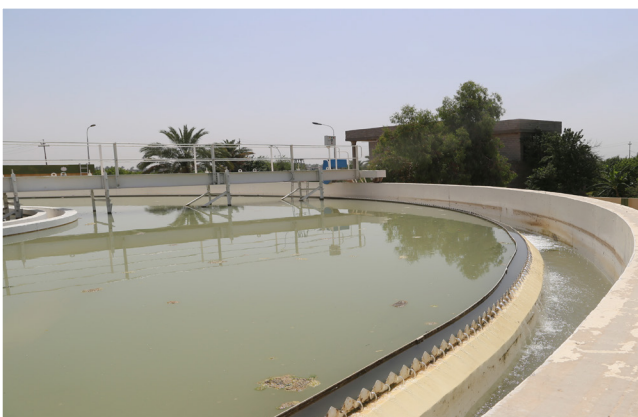
Rehabilitated Sedimentation Tank
