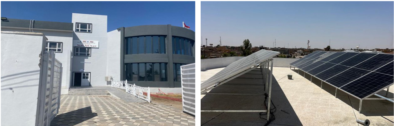
Rehabilitation of Hawija Municipal Building in Hawija, Kirkuk
