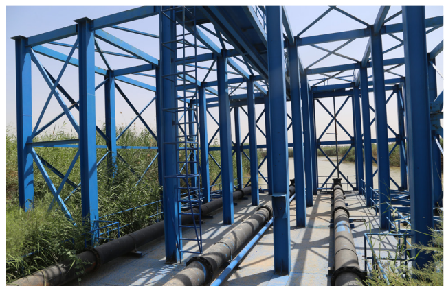
Rehabilitated Intake Structure
