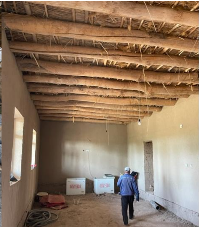
Picture 6: Locally used construction timber in Karakalpakstan, Puttkamer 2022
