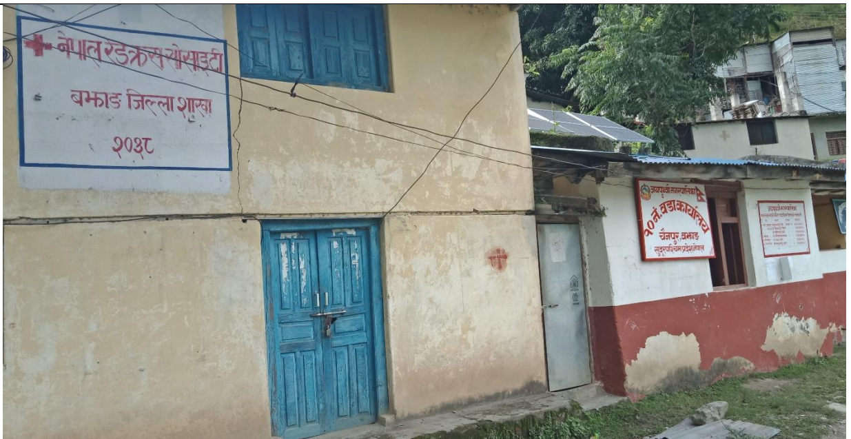
Figure 13 Safety walk - ward office near Nepal Red Cross Society, Bajhang, Jayaprithvi
