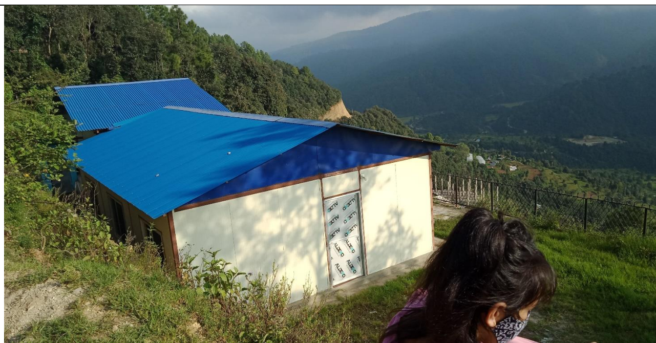
Figure 33 Safety Walk - safe house- (no survivor at that time), Amarghadi
