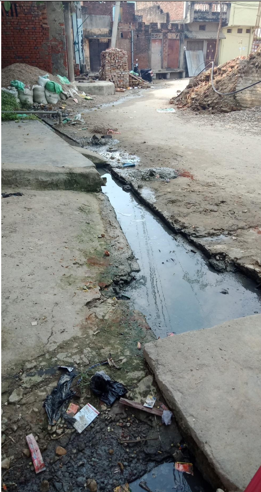
Figure 10 Drainage System in Eklaini Bajar, Nepalgunj
