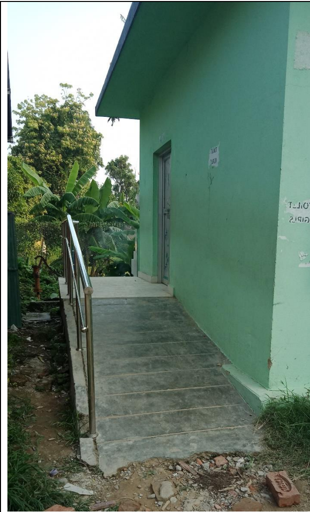
Figure 22 Toilet with ramp in school, Dhangadhi
