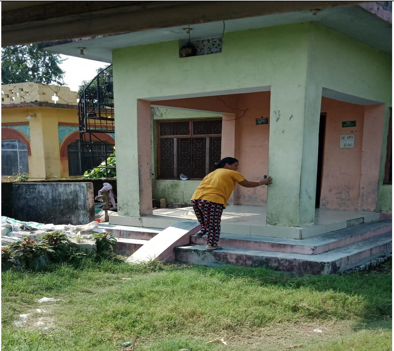
Figure 9 Respondent (PWD) facing difficulty to climb stair in her rented house, Dhangadhi
