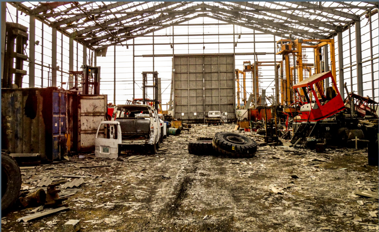
Figure 3: Workshop before rehabilitation
