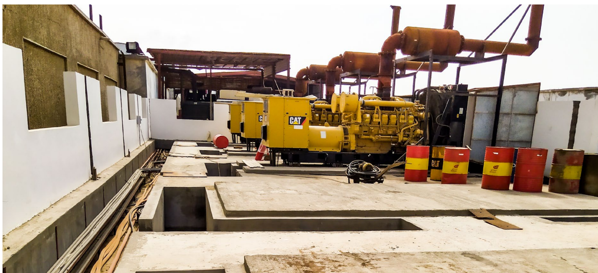
Figure 1: Generator shelter before rehabilitation
