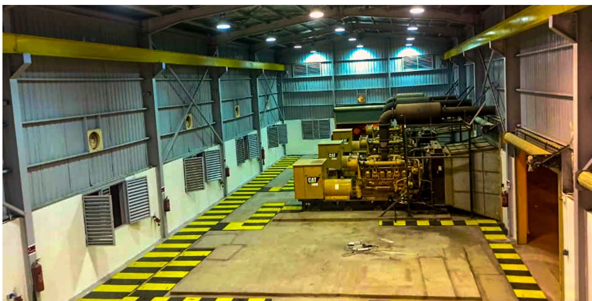
Figure 2: Generator shelter after rehabilitation
