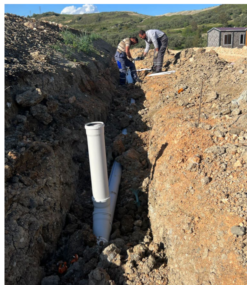
Installation of pipes for waste water at Hatay container city
