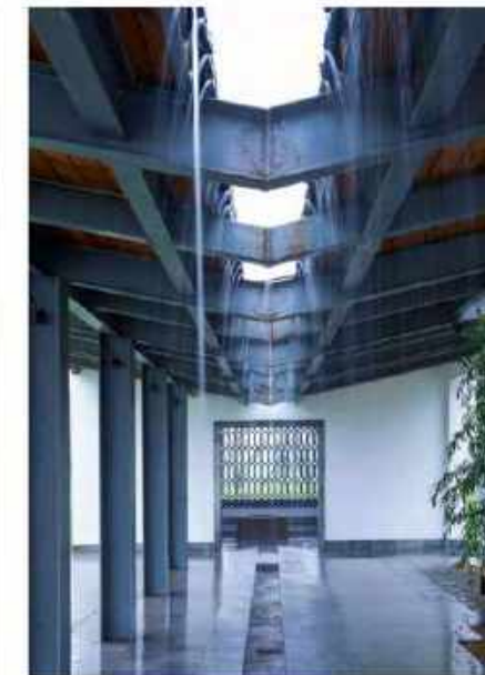
Rain-hearing Pavilion, 2019, Hefei, TJAD architects
