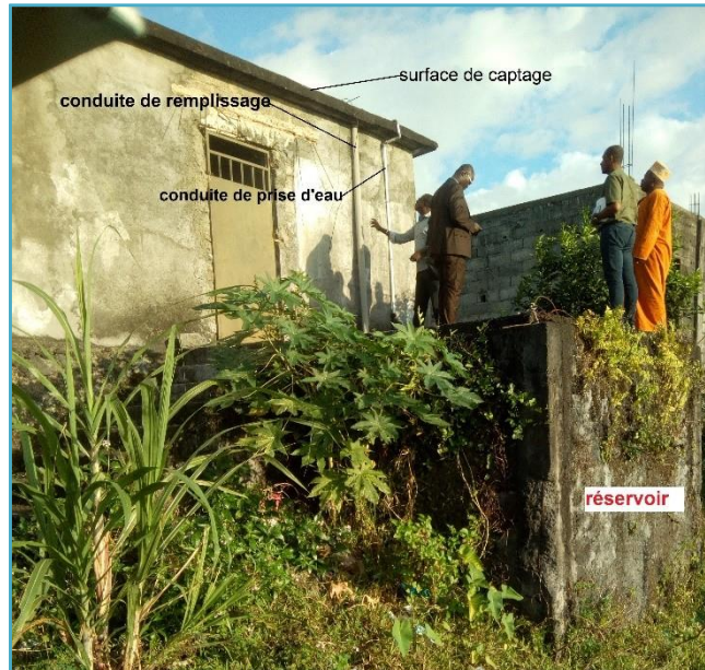
Photo 1: Concrete tank in Mkazi
