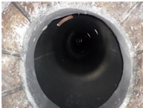
Installation of mullite-based castable in a rotary kiln
