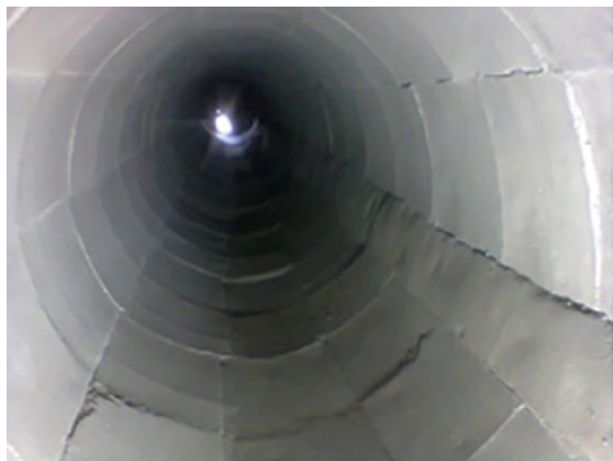
Kiln interiors lined with mullite-based casting
