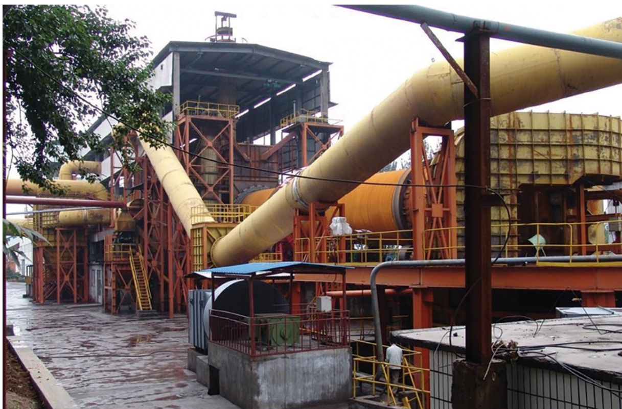
A typical pelletization plant
