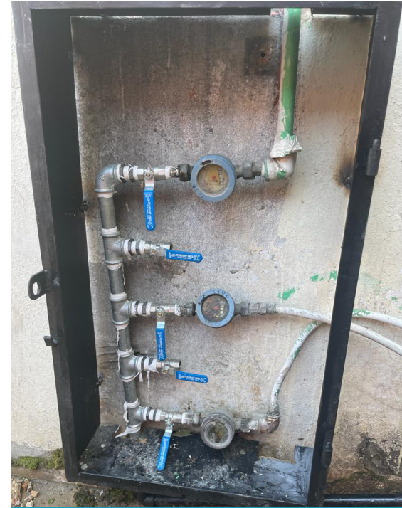
Replaced water manifolds and meters
