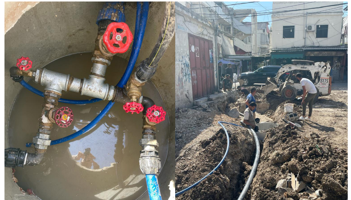
Installed PVC water pipes and connections
