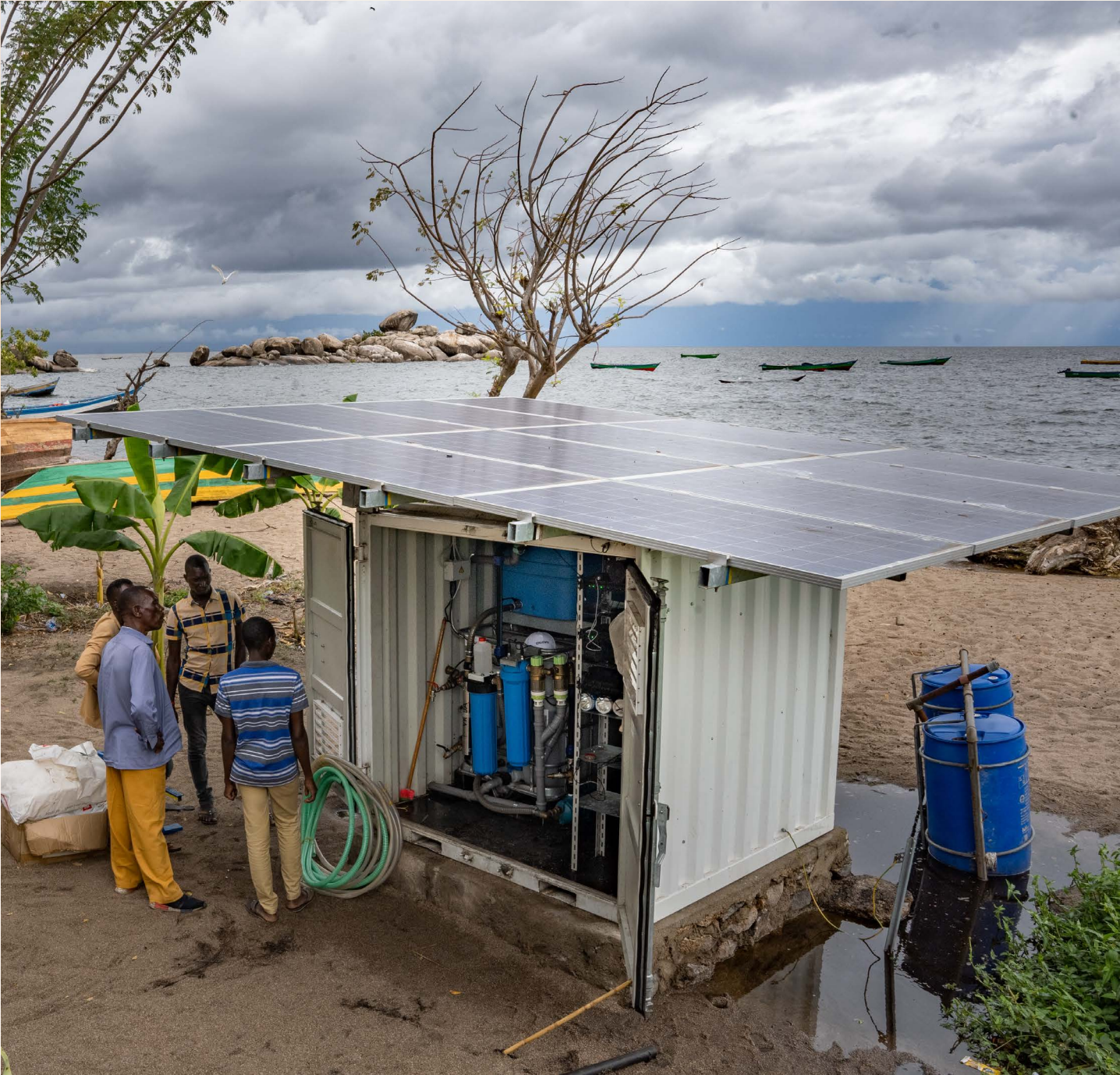
OFFGRID BOX technology, a system that uses solar power to produce electricity and clean, safe water in one shipping container and can convert sunrays into renewable electricity.
