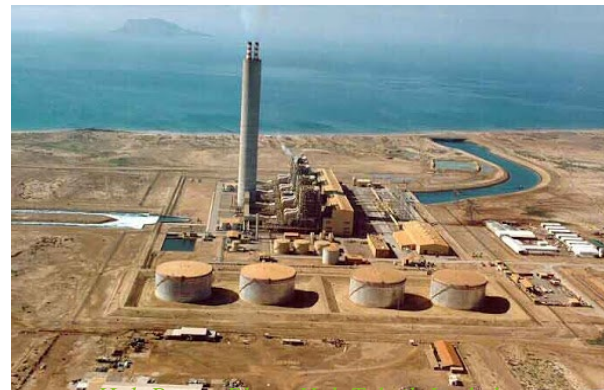
Hub Power Plant, Hub Tehsil, Lasbela
