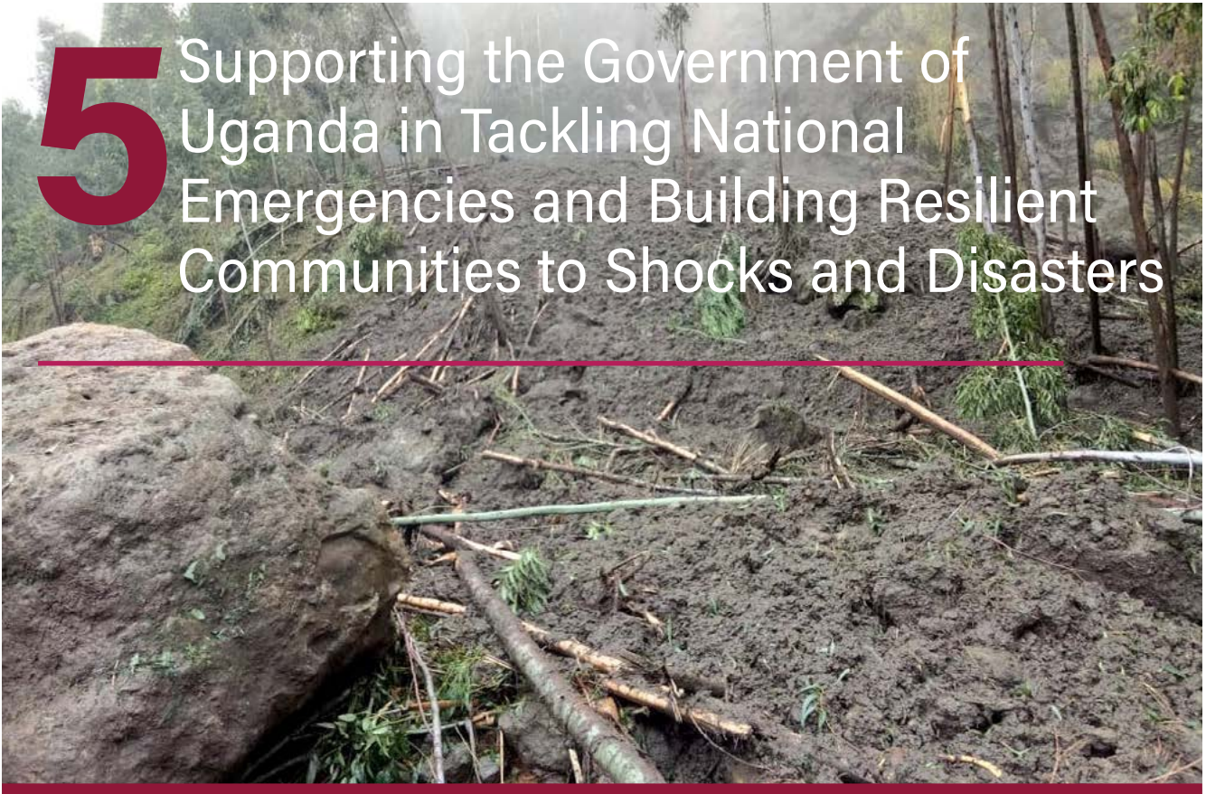
PHOTO: Mudslides proved devastating along Mbale-Nkokonjeru Road in Eastern Uganda. ©Uganda National Roads Authority
