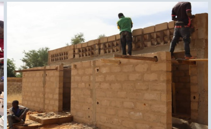
Image construction of latrines in Seytenga (December 2022)
