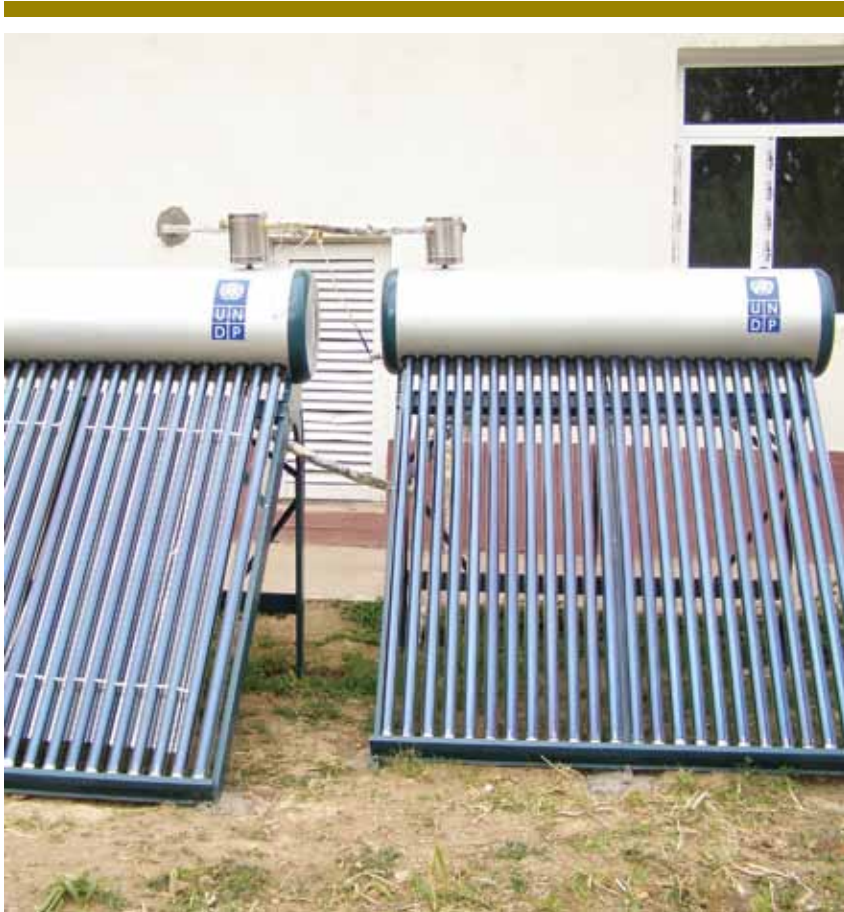
Photo 6. A solar water heating system, installed at the “Baymukhamedov” rural health clinic .
