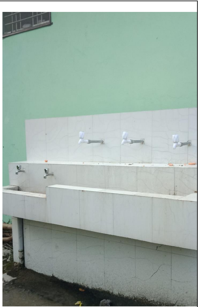
Figure 23 Figure children friendly water tap in school, Dhangadhi
