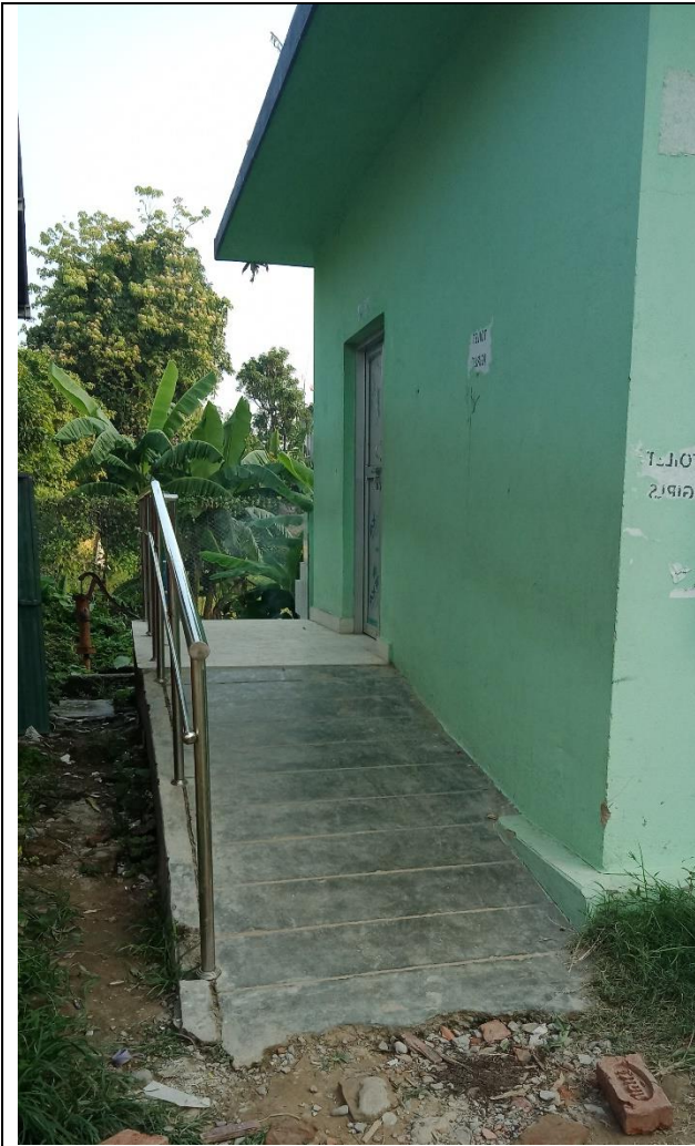
Figure 22 Toilet with ramp in school, Dhangadhi
