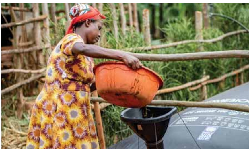
Mukagikwiye Viviane inserting organic waste into the digester via the inlet sink 4.
