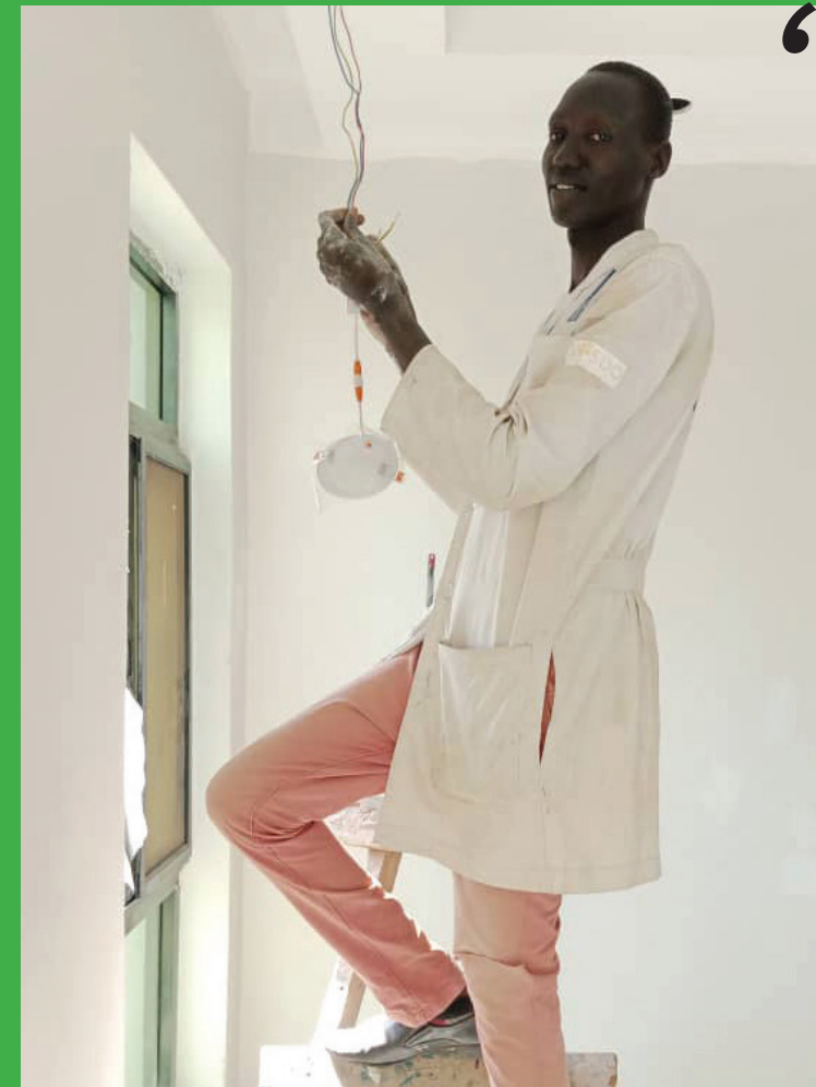
Elijah Ngor Anok making electrical repairs, 2021.
