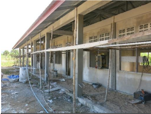
School classrooms being constructed on cleared ground in Ban Thongsaen, Bolikhaxai
