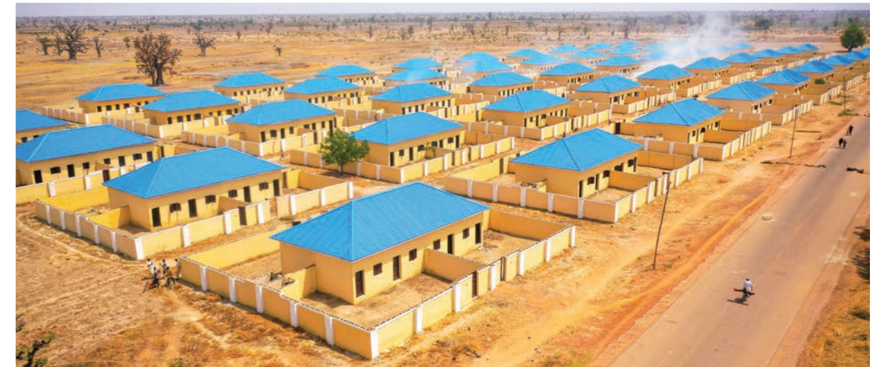
500 2-bedroom units were constructed in Banki
