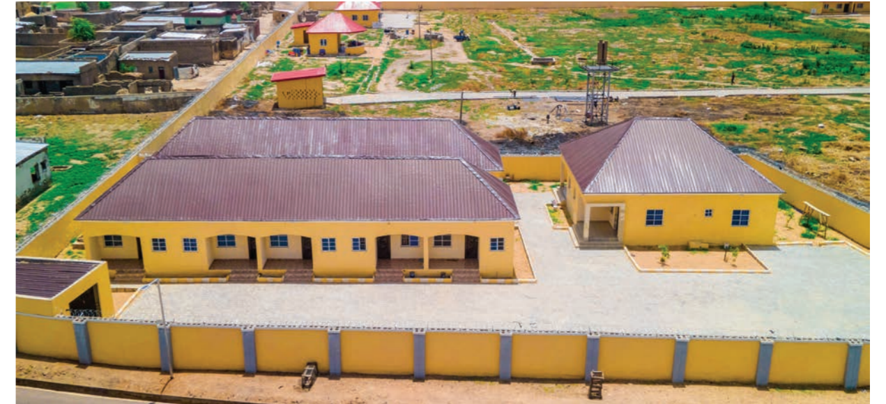
Residence of immigration officers constructed in Banki
