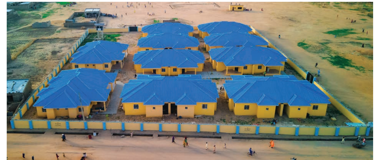
Constructed teachers quarters in Banki
