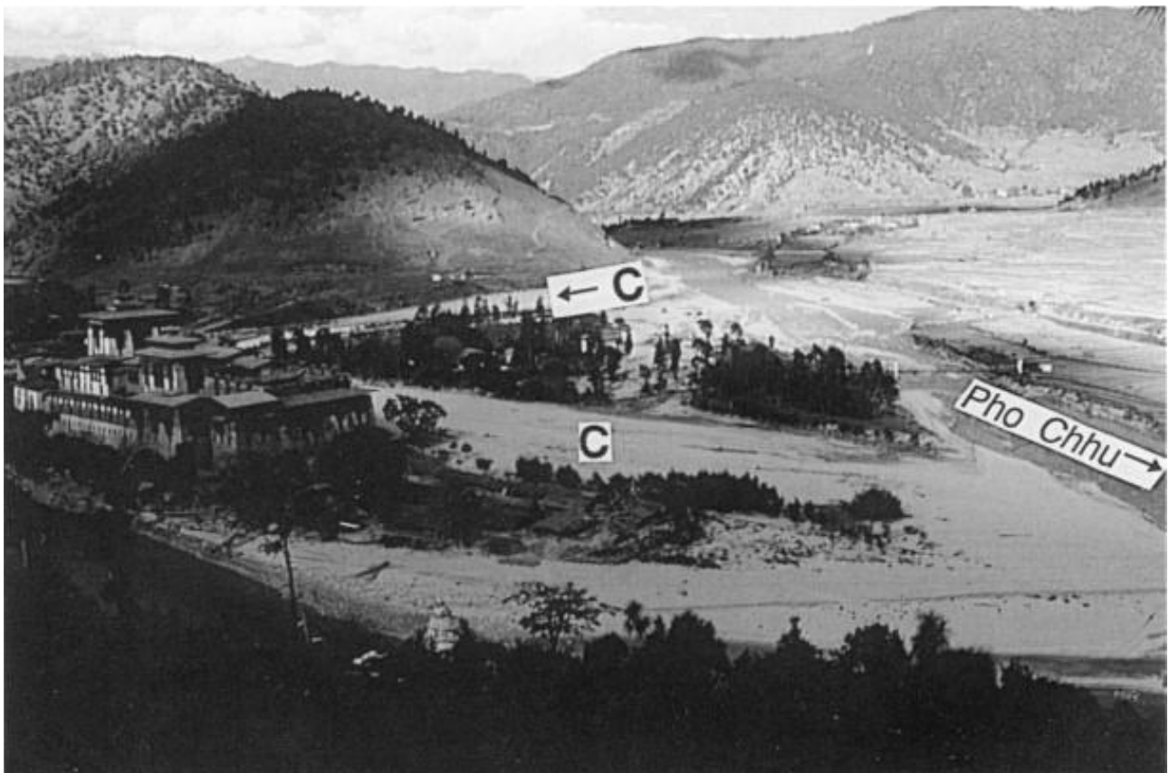
Figure 2. Flood damage in and around Punakha dzong due to Lugge Tso GLOF (6 & 7 October 1994), sourced from Watanbe & Rothacher (1996)
