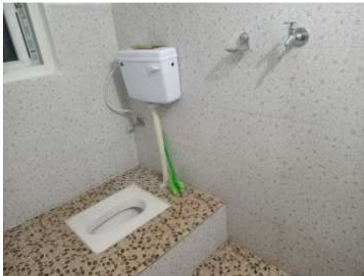
Fig: Internal plumbing and fitting in toilet
