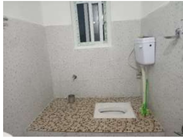
Fig: Internal finishing of toilet
