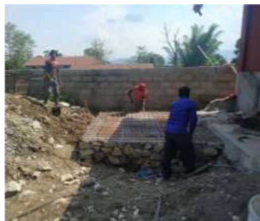
Fig: Construction of septic tank
