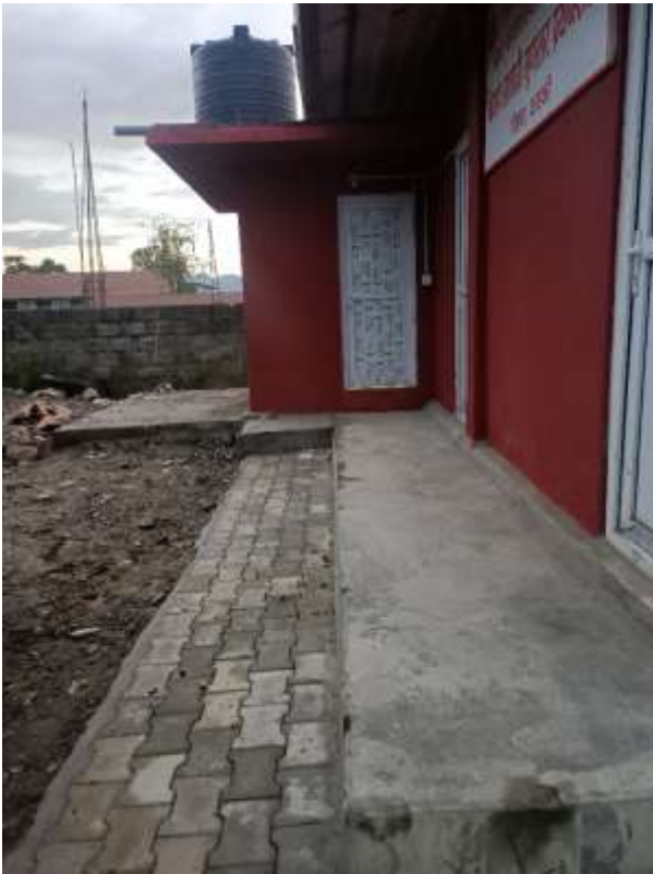
Fig: Use of plastic-mix pavement tiles
