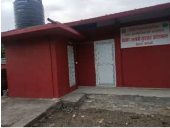
Fig: Completion of toilet
