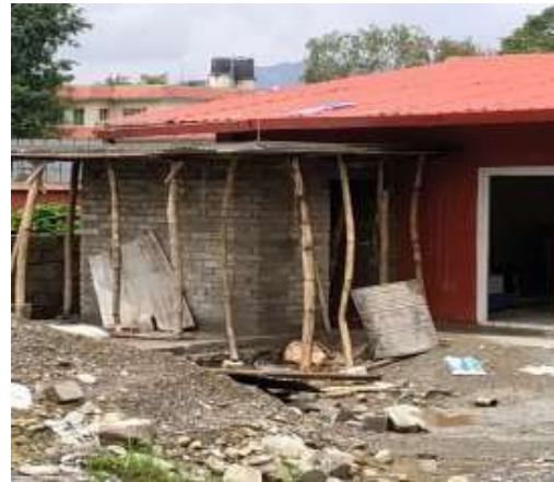
Fig: Construction of toilet structure
