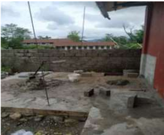
Fig: Construction of safety tank
