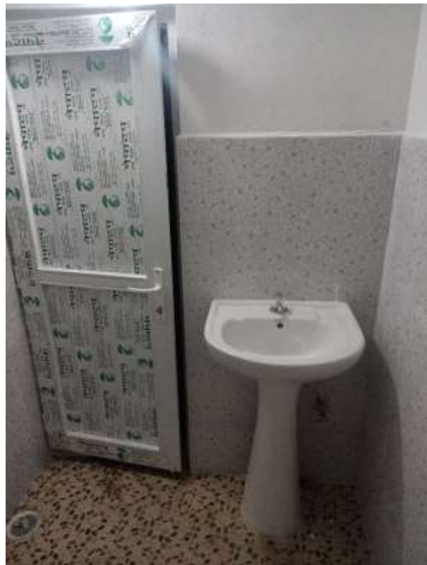
Fig: Use of basin in internal part of toilet
