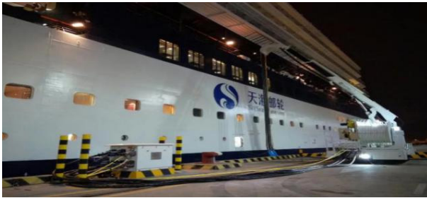
Figure 7-4 Shore power ship connection at the Prince Bay Cruise Homeport
