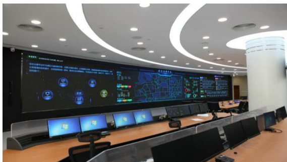
Figure 7-9 Smart City Command Center Hall, Futian District, Shenzhen
