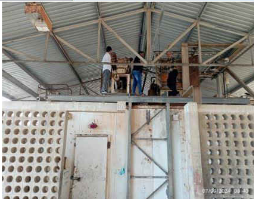
Figure 5 Photos Showing subproject situation in Fuqm area
