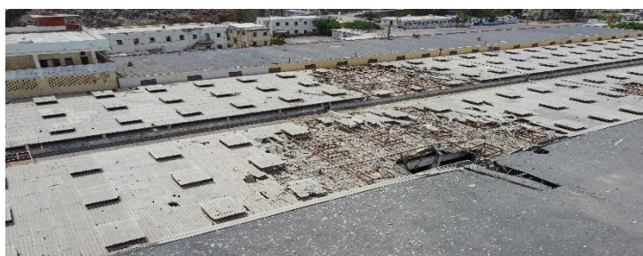
Figure 2. Asbestos Cement Sheets
