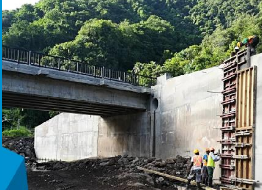
Reconstruction of Cumberland Bridge © UNOPS
