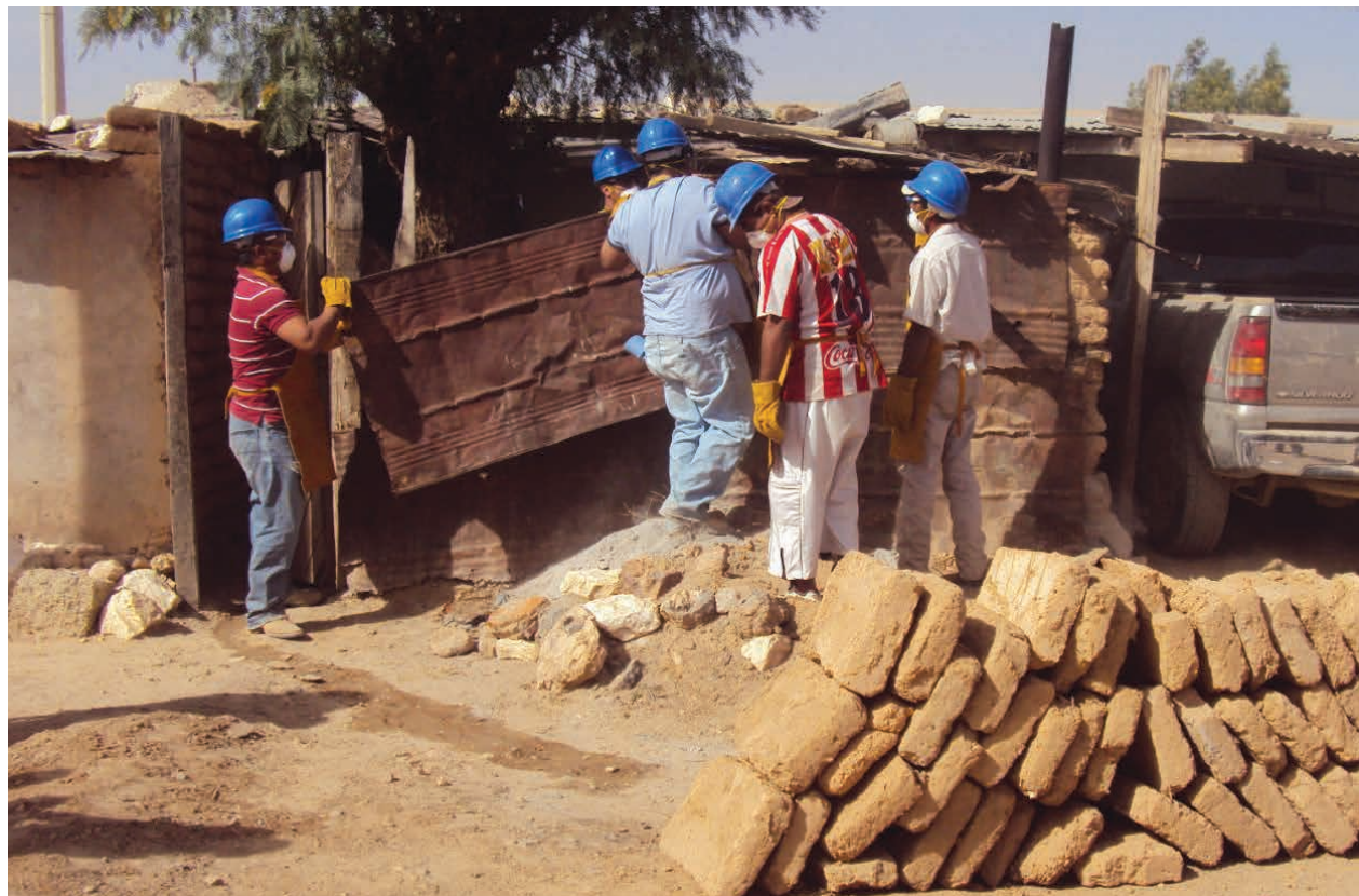
UNDP-GEF project removing recycled PCB-containing materials used as building material in a community in San Felipe Nuevo Mercurio, Mexico.
