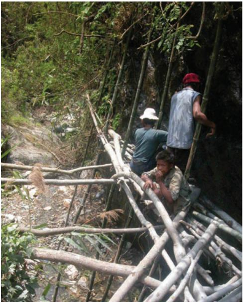
Bamboo scaffolding enables community members to cut into rock, during the construction of the micro-hydropower installation.
