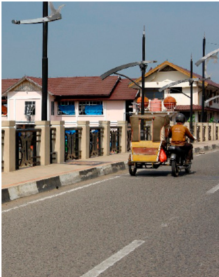
Photo: Peunayong bridge after rubble and debris clearance activities were complete. Faisal Ridwan/UNDP Indonesia
