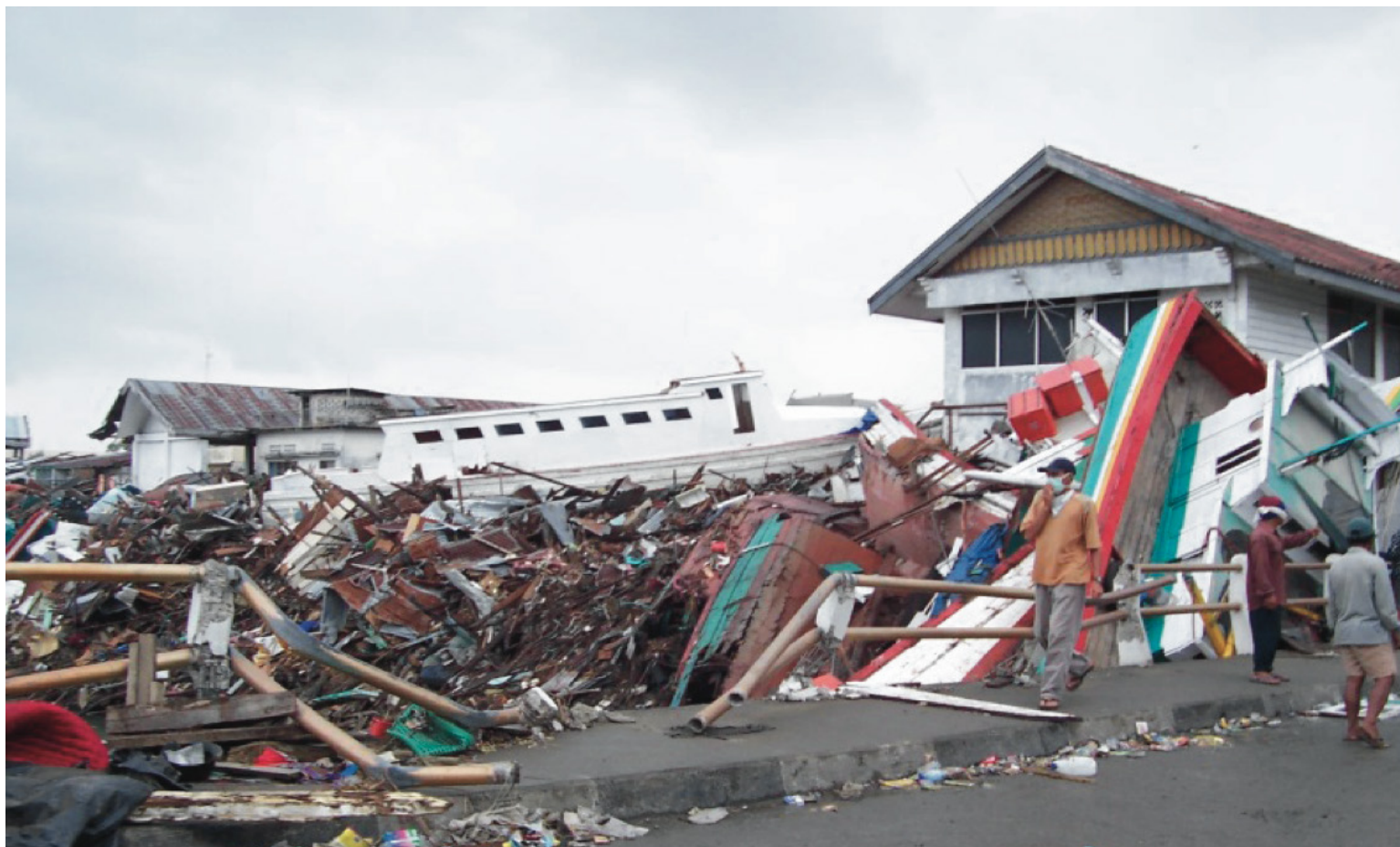
The 2004 Asian Tsunami killed approximately 230,000 people, about half of whom were in Aceh, Indonesia. This bridge in Peunayong, Banda Aceh, was covered in debris. Photo: Faisal Ridwan/UNDP Indonesia
