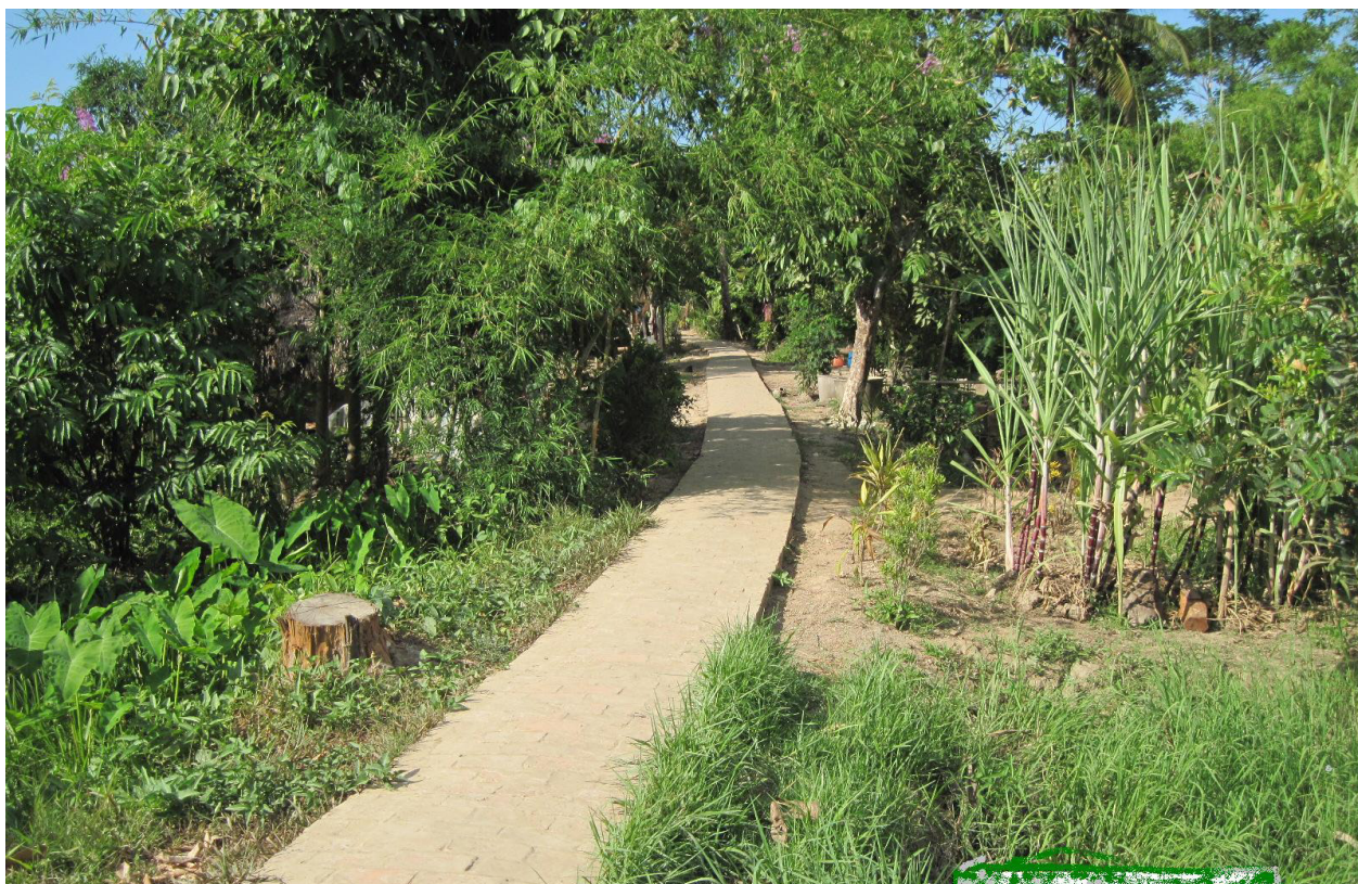
UNDP's 'build back better' approach in Myanmar helped Chaung Ma Gyi village improve on pre-Cyclone Nargis facilities: a mud path which was prone to flooding is now elevated and paved. Photo credit: UNDP Myanmar
