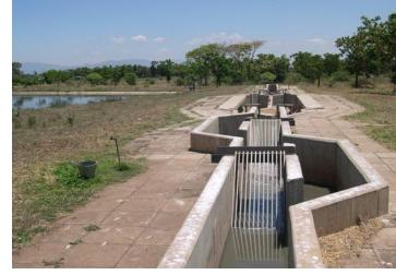
key components: (1) treating of waste water through waste water stabilization ponds, (2) releasing treated waste water from maturation ponds through trapezoidal channels to farmlands, (3) clearing and demarcating farm plots adjoining the oxidation ponds for new farms, (4) changing the mindset of farmers on the suitability of odorless waste water for agricultural production, and (5) establishing a farmers association, complete with leadership structures for aggressive market access.
